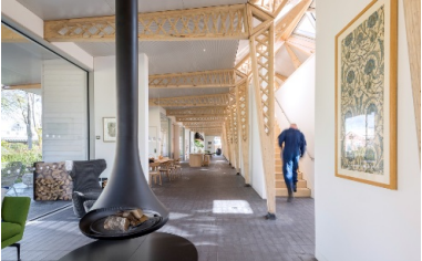
Close-up of the roof construction
