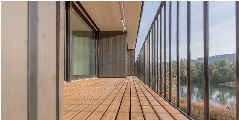
View of Bildweiher with generous balconies
