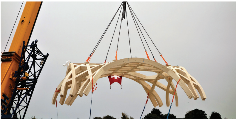
Blumer Lehmann's expertise in Free Form timber was used to create arabesque branches that curve and weave into a canopy of geometric designs.
