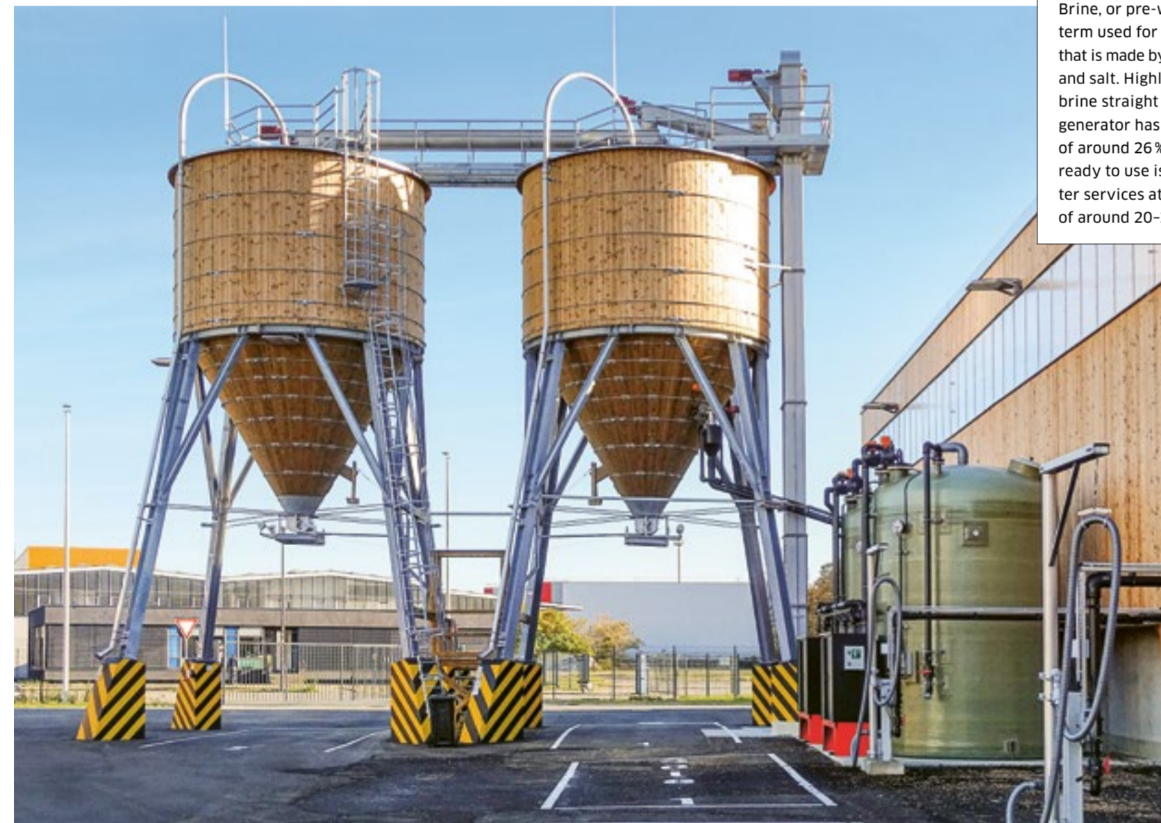
Silo and brine facilities, works and construction yard, AWB in Cologne
